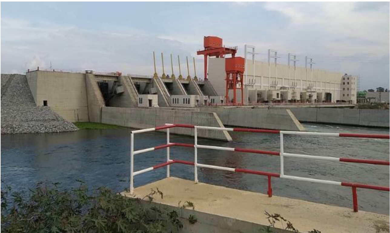
Figure 1: 183 MW Isimba hydroelectric power station.
